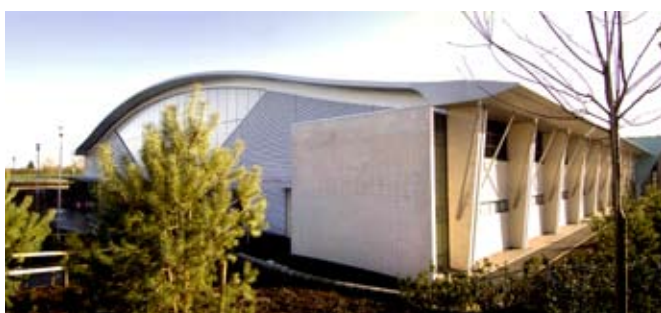
High Performance Centre at Jordanstown £2,977K
